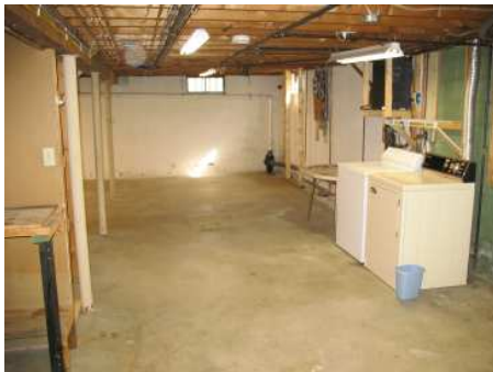
Basement Wash area
